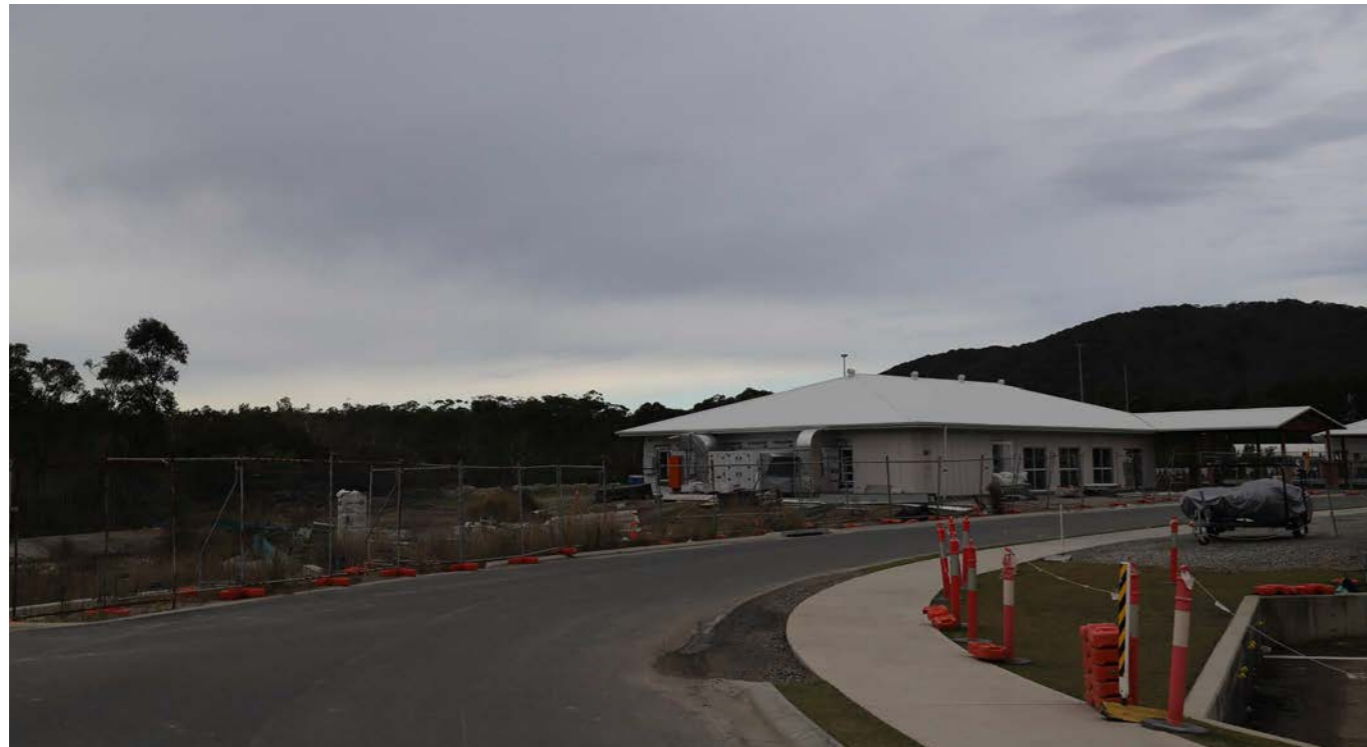
Photo 15. VP12 - View east-north-east towards the site from Royal Pines Parade.
